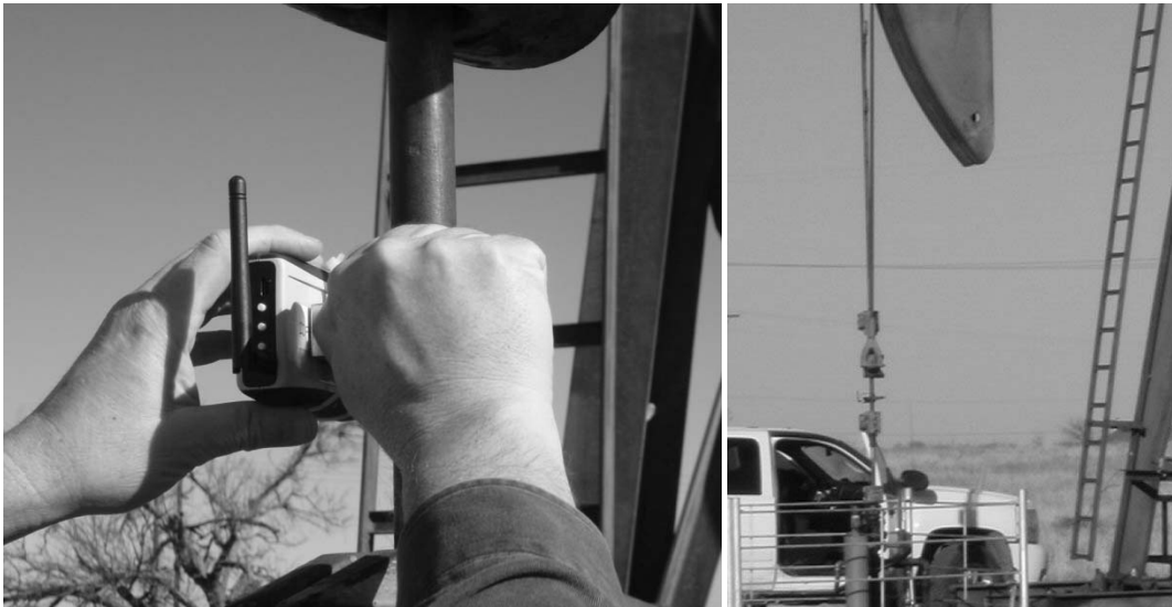
Figure 2 – Wireless Polished Rod Transducer (WPRT) Installation
